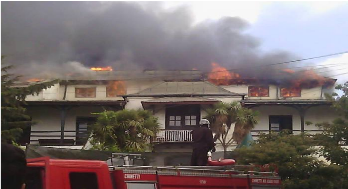
Addis Ababa's iconic Taitu Hotel burned to the ground; it took firefighters over 1 hour to arrive even though they were stationed only 5 minutes away. The 108-year old Taitu Hotel was burned beyond repair (sustained 75% damage) while fire fighters stood idly by until it was too late, despite the claim by the government that the fire was controlled quickly
